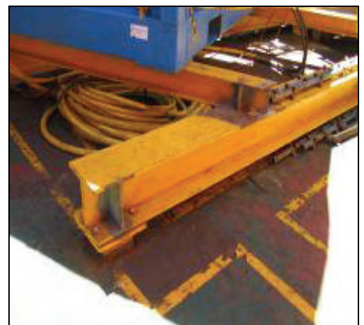
Figure 5 – Equipment placed on designated escape route
