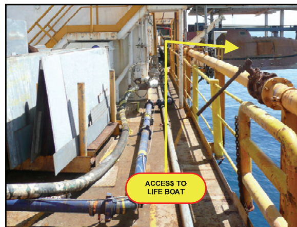
Figures 1 & 2 – Flow lines run along designated escape routes
