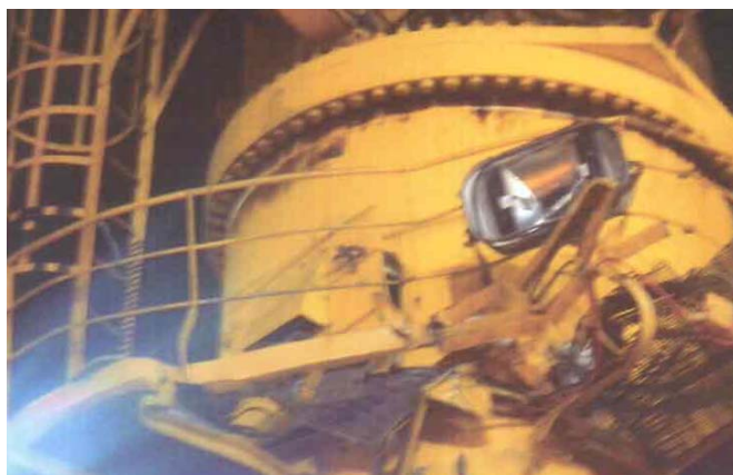
Damage to crane walkway and light caused by impact of swinging block.
