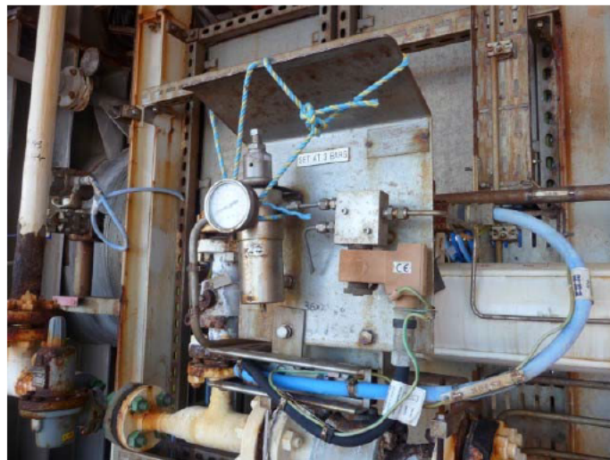
Figure 1 - Instrument Air Tubing Arrangement
