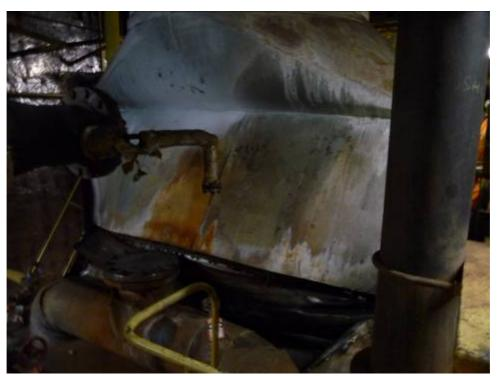
Damaged boiler exhaust uptake
