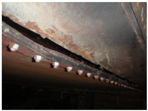
Furnace casing damage
